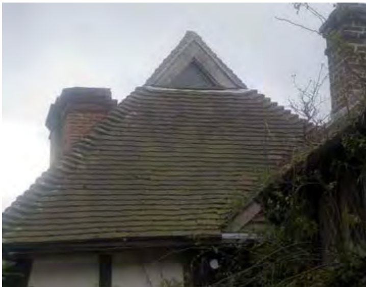
Figure 8: Example of a 'Gablet' in Shipley Parish
