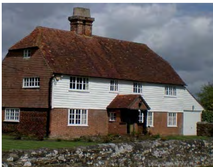
Figure 11: Example of 'weatherboarding' in the Parish
