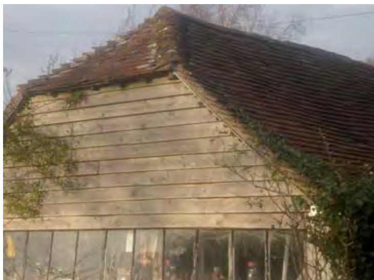
Figure 5: Example of 'Partial Hip' roof
